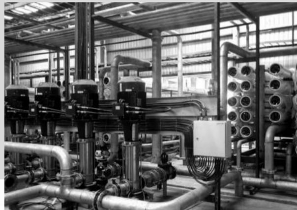
11 MLD Zero Liquid Discharge system at Hawassa Industrial Park, Awasa, Ethiopia
